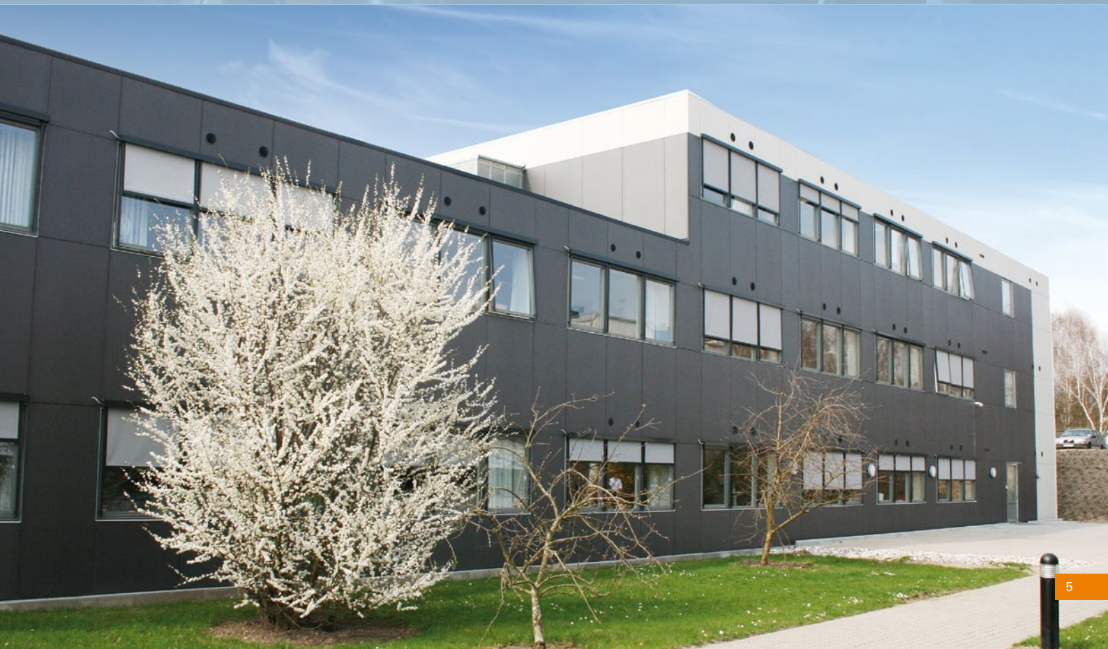
The office building from the outside. Intake and exhaust pass through the facade covered by a facade grille.
